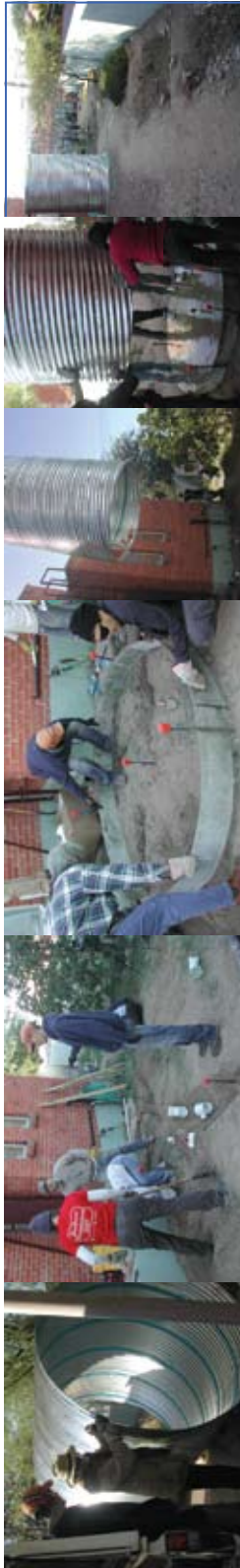
Installation of a water rain collection cistern with community volunteers, funded by the Blue Water Project Grant.
